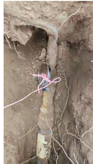
Figure 3-2: Examples of Copper Pipe, Lead Pipe, and Galvanized Pipe
